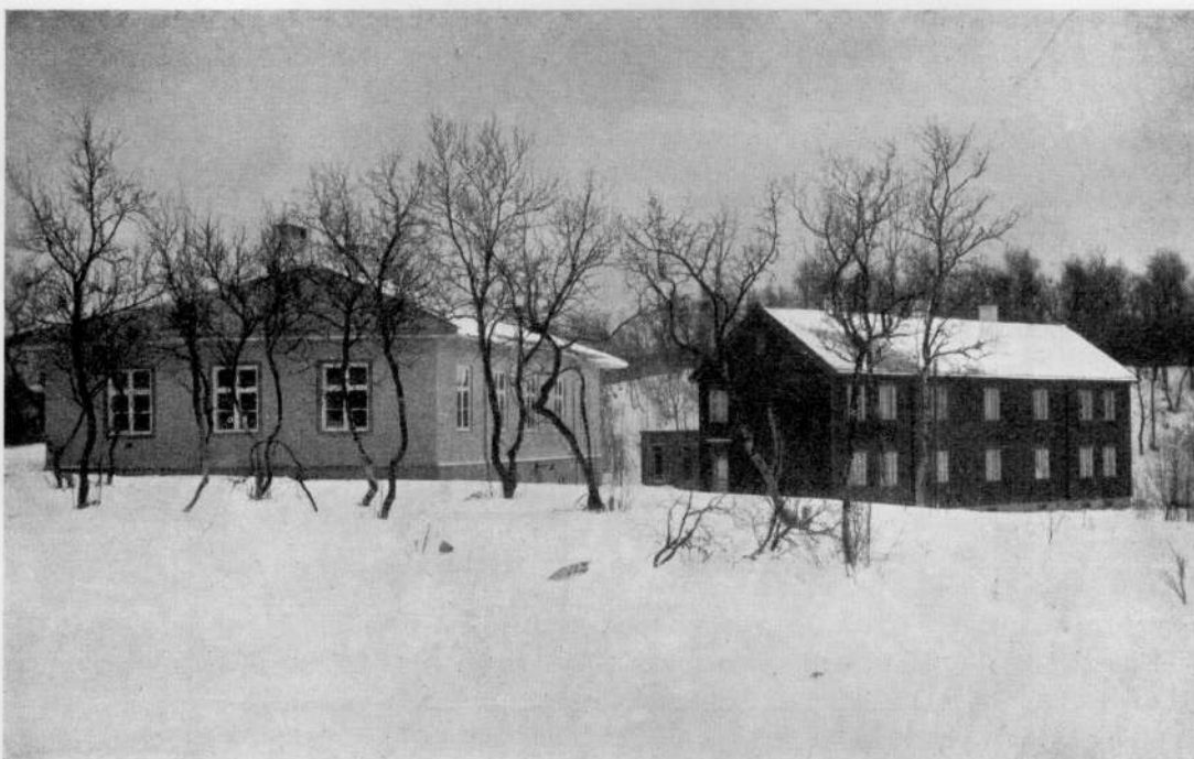
Fig. 8. The main observatory and dwelling house. View from S—W.
